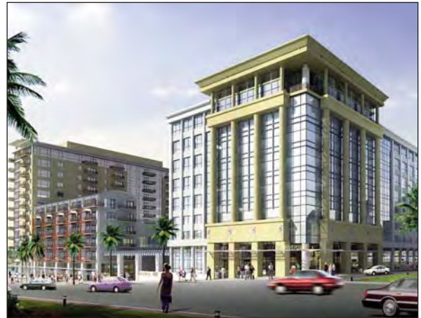
Elkins will obtain LEED Silver certification for its new corporate headquarters in Jacksonville.
